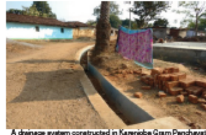
A drainage system constructed in Keresjuba Gram Panchayat
