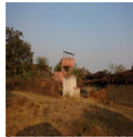
Community water tank constructed during first tenure of Ashren Kerkatta
